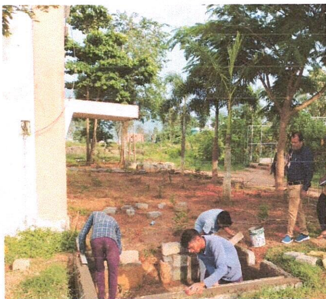
Water Harvesting Pit during Construction
